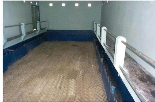
Submerged aerobic biofilter
